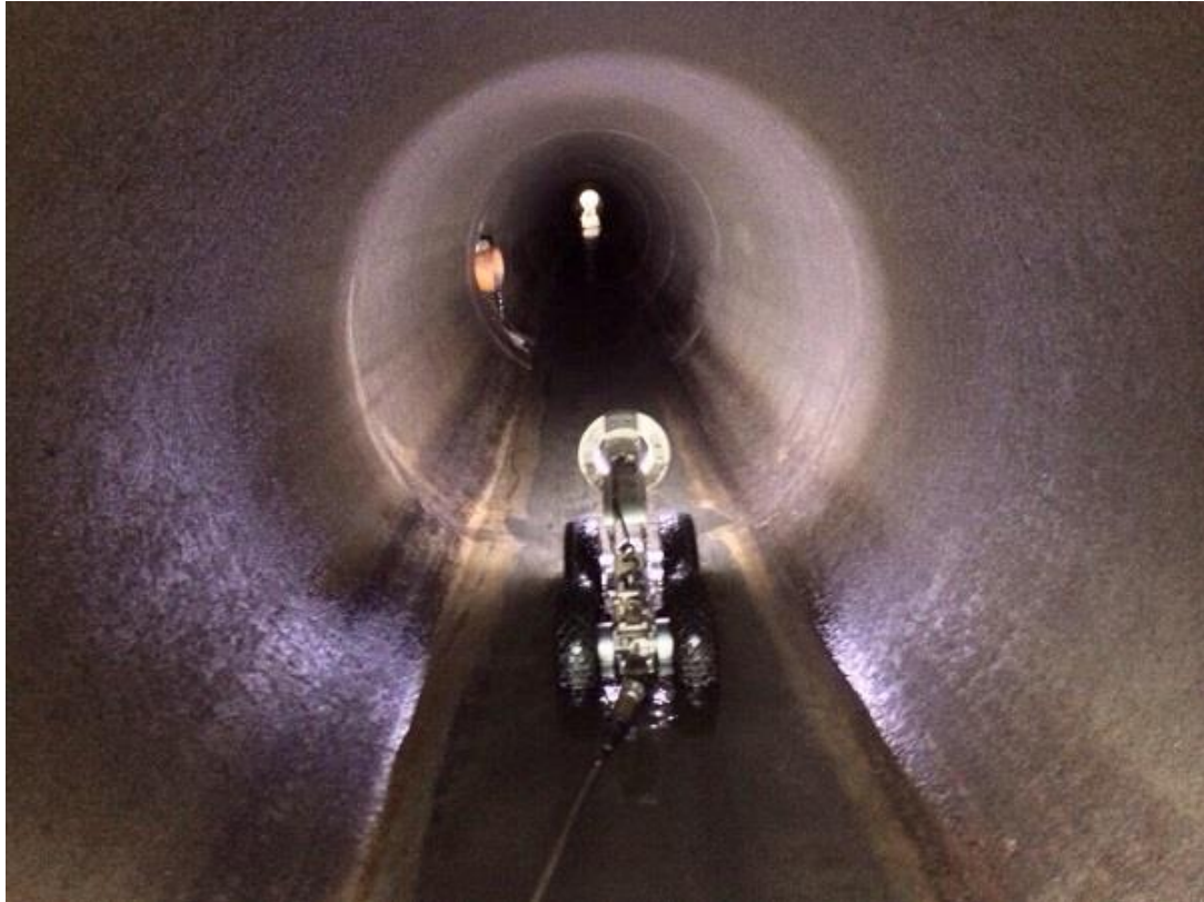
Figure 3, Sewer Pipeline CCTV Inspection
