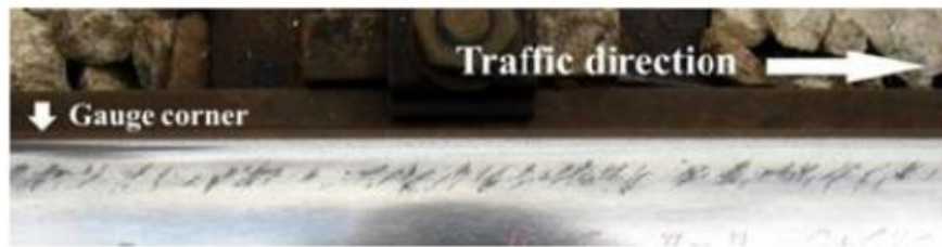
Figure 3. An RCF defect [5].
