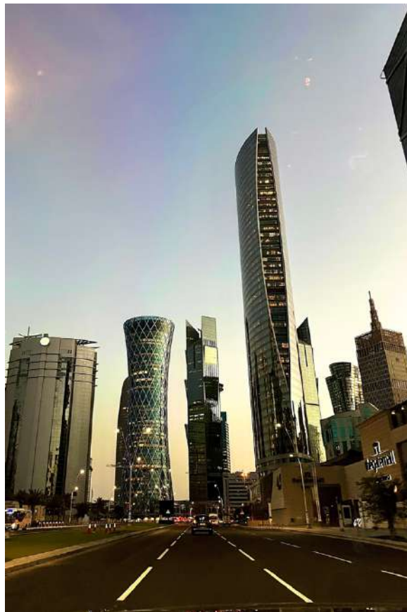
Figure 36. The application of tinted glass and reflective materials in towers in West Bay. Source: Author.
