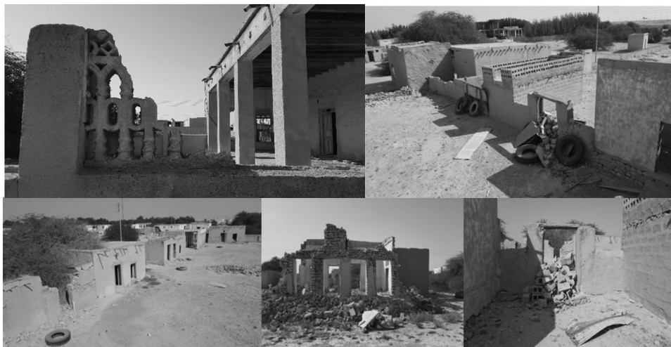
Figure 4. Shows several views of the village's current condition.
