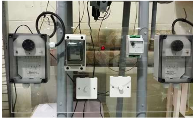
Figure 19 - Control board components installation
