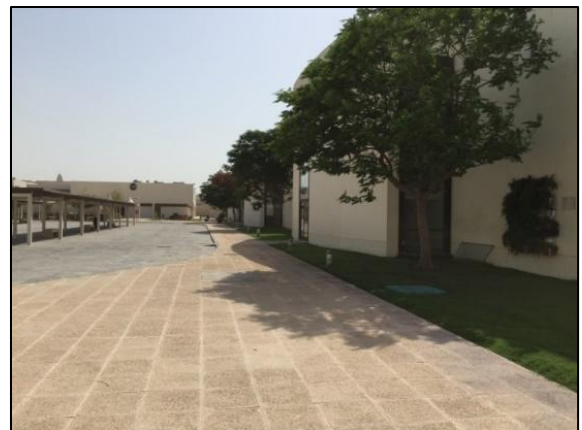
Figure 20. Exposed Walkway of the Women’s Engineering Building
