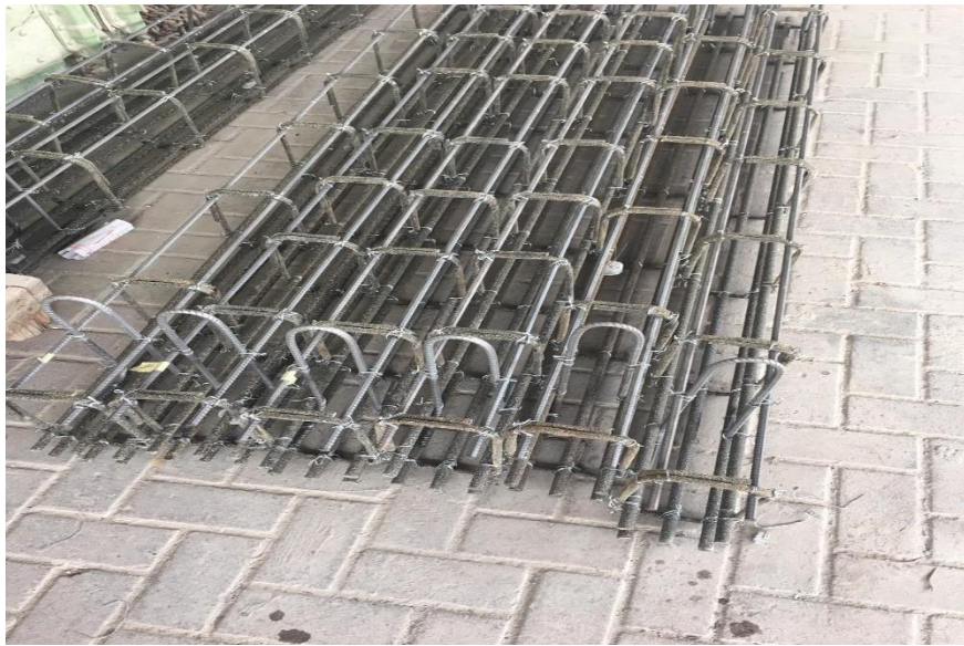
Figure 18. Assembly of the reinforcement cages
