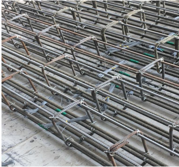
Figure 19. Installation of the strain gauges for the BFRP bars.
