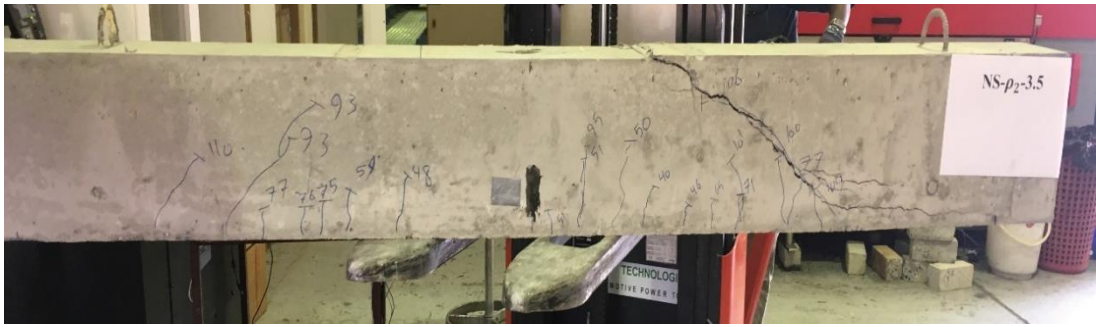
Figure 47. Beam B-12 Shear tension failure.
