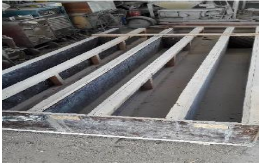
Figure 17. Shuttering used to cast beams
