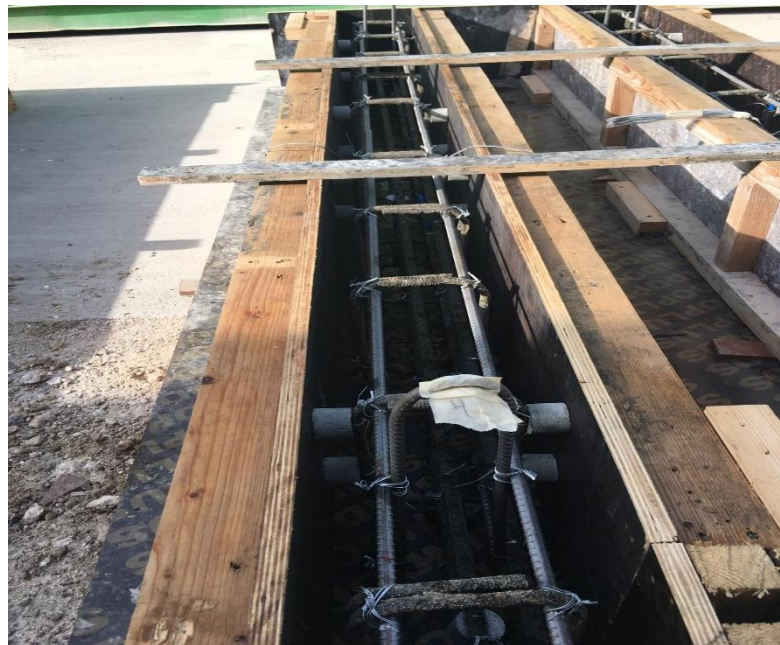
Figure 20. Installing Reinforcement cages in the shuttering.
