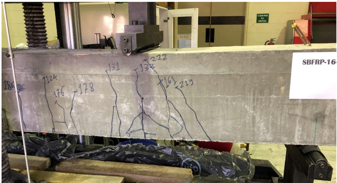
Figure 63: Cracking pattern of beam 9 (SBFRP-16-1200)
