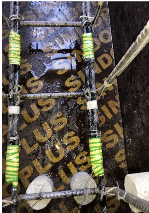
Figure 13: Typical spliced FRP bars before casting
