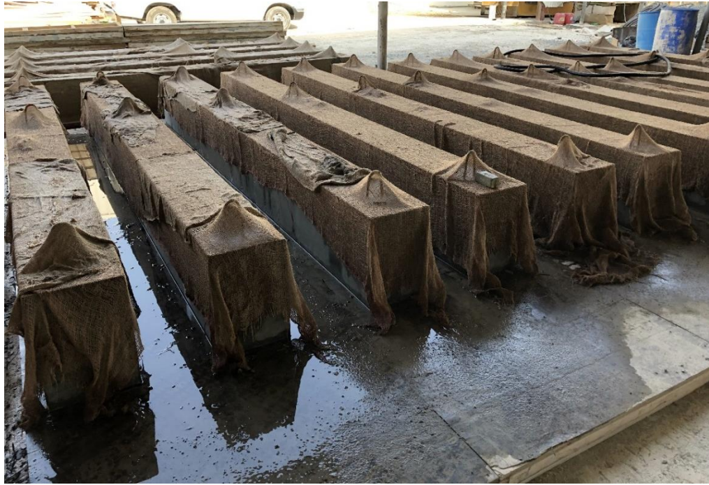
Figure 16: Curing of the beams
