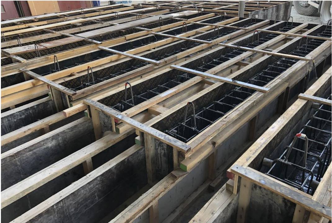
Figure 14: Spliced beams before casting
