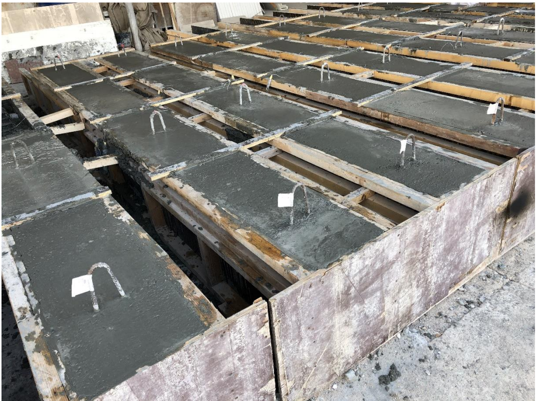
Figure 15: Casted concrete beams
