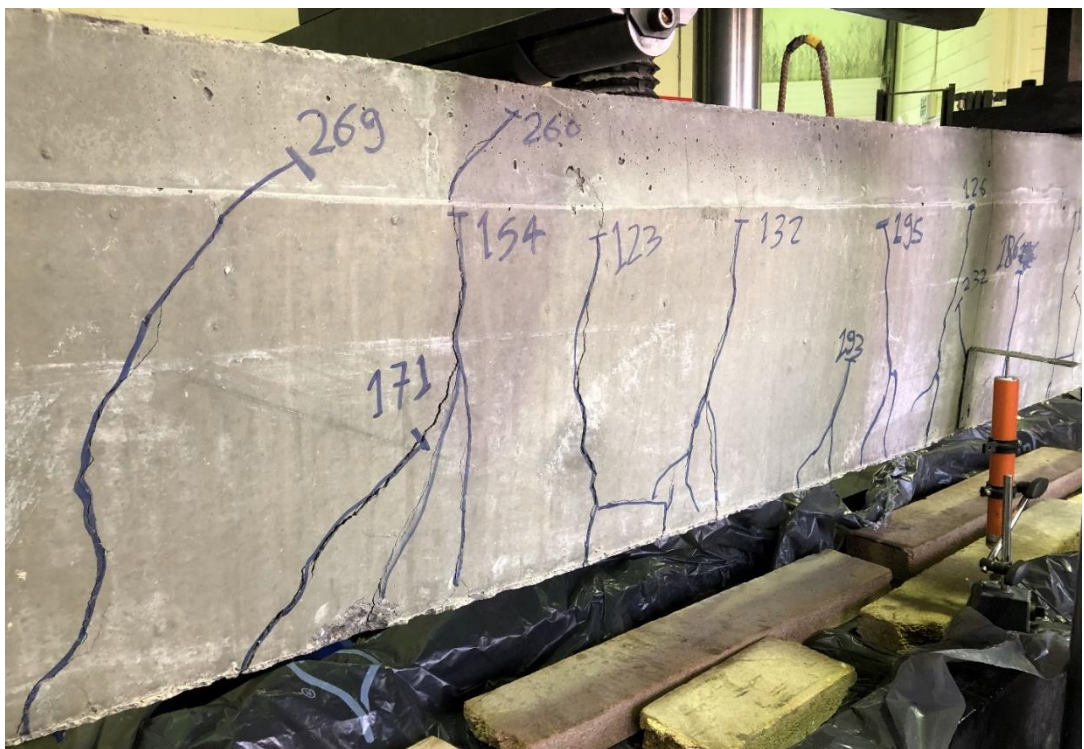
Figure 64: Cracking pattern of beam 9 (SBFRP-16-1200)
