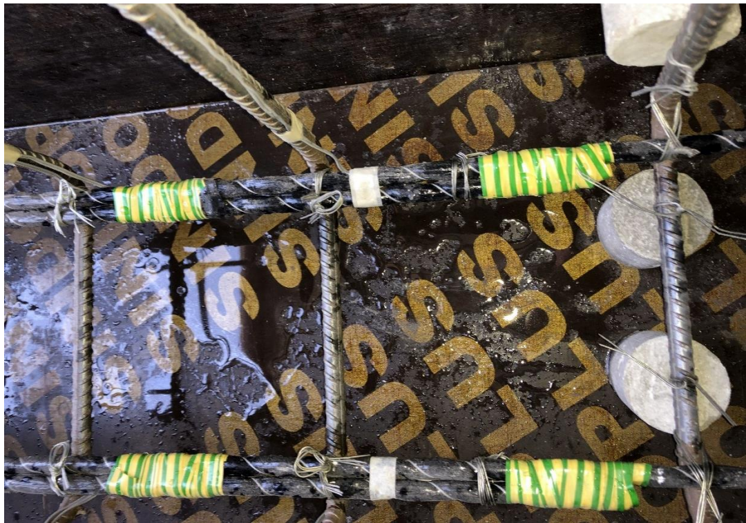
Figure 20: Installation of strain gauges
