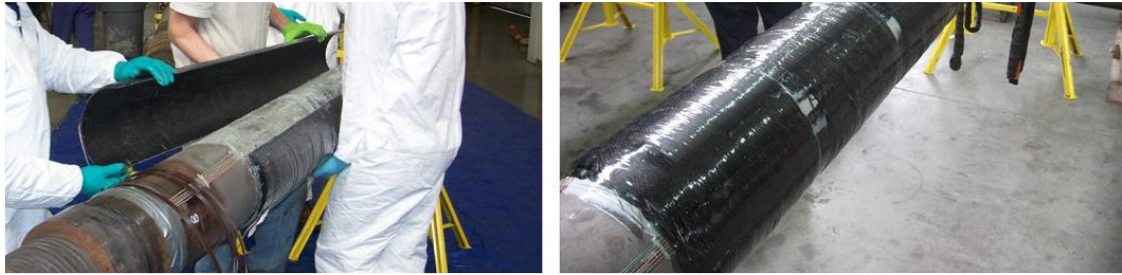
Figure 36. Installation of the carbon half-shells [129].
