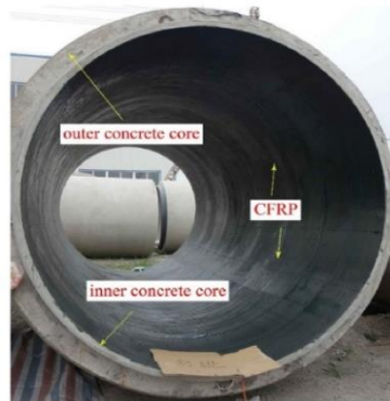
Figure 31. Prepared CFRP-lined PCCP before assembly [114].
