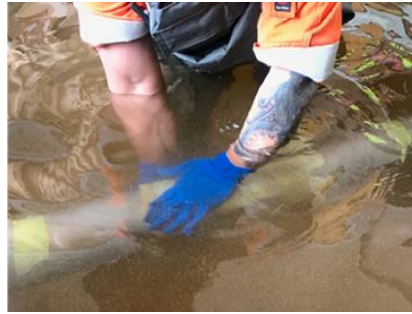
Figure 13. Repairing in water with hybrid glass/carbon layers [50].
