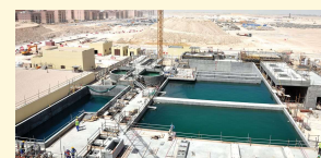
Wastewater Treatment Plant in Qatar
