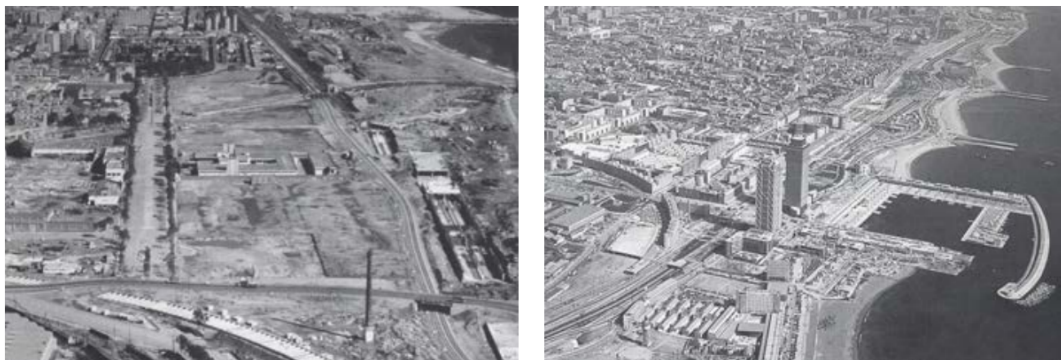
Figure 3: Photographs of Barcelona Sea Front before and after 1992 (Busquets, J. 2005)
