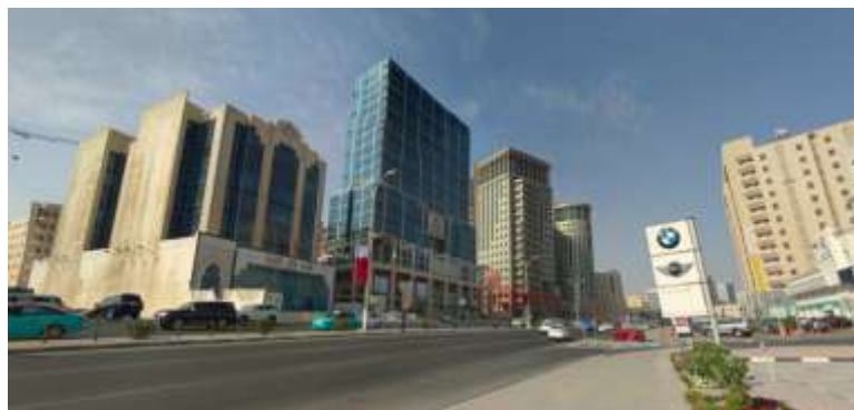
Fig-16: Doha's high-rise commercial buildings
