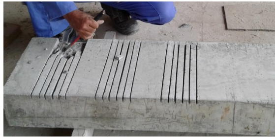
(b) Removal of the concrete.
