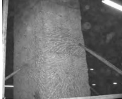
a) Chipping of existing column face
