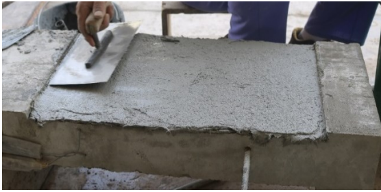
a) Application of first layer of mortar
