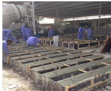
(b) Concrete casting and concrete surface finishing.
