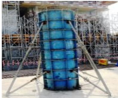
c) Formwork installation and casting concrete
