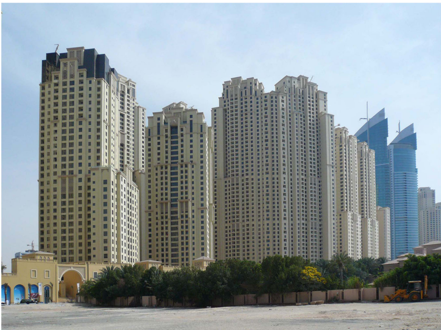
Fig. 1 Residential high-rises in Dubai (source: authors)
