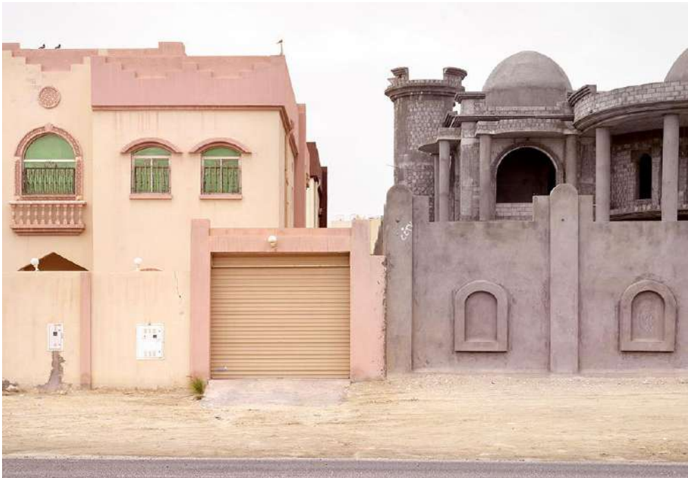
Figure 23: Houses Built and Under-Construction in Al Gharrafa District, Doha. Source (Elblaus, 2017)
