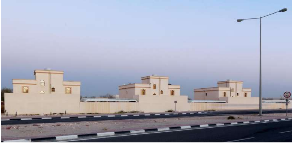
Figure 22: A Typical Alignment of Modern Neighbourhoods in Doha, Bani Hajer District. Source (Elblaus, 2017)
