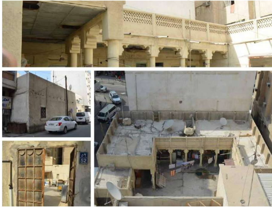
Figure 21: Recent Situation of an Old Courtyard House in Doha. Source (PEO, 2015)
