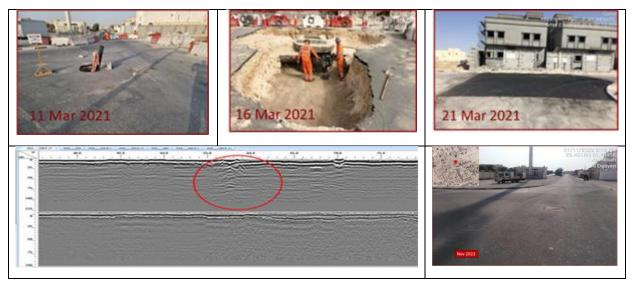
Fig. 6: Different stages of sinkhole evaluation and repair – Case Study 1
